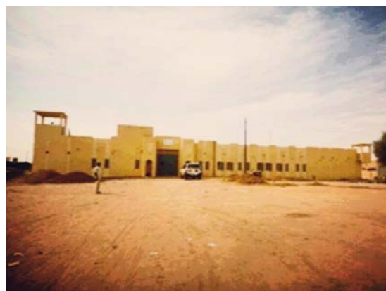
La Maison d'Arret et de Correction de Gao, Mali, after refurbishment, July 2014.
